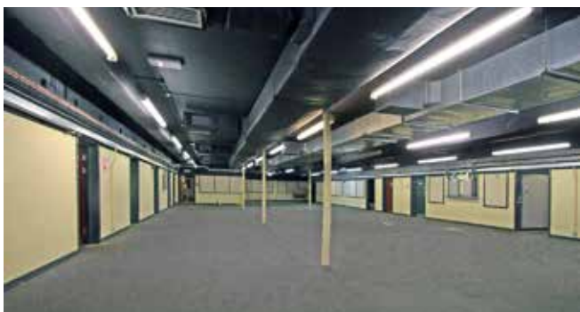
One of the large open-plan rooms on the upper floor. This view is from February 2011 when the lights were still working. Photo Nick Catford
